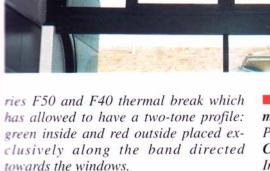
The large curtain walls with the curved glass components (the 'glassfall') have been obtained using the system W50 by Alcoa, whereas the internal railings have been made from the system GR 14 by Alcoa and painted in the same aqua green shade"
